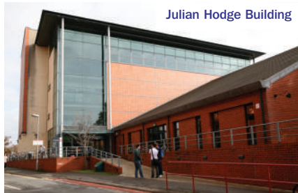
Julian Hodge Building
